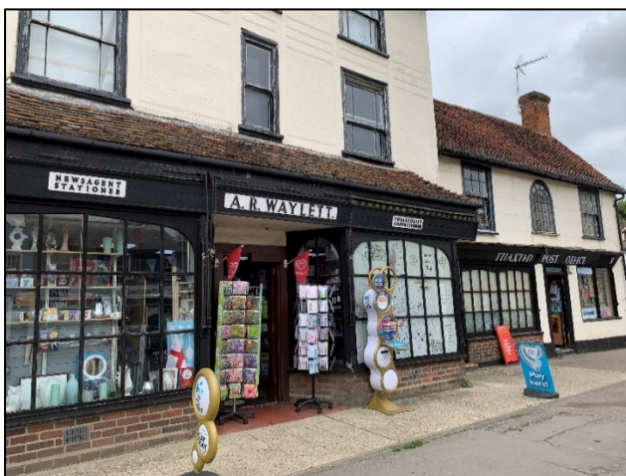
Attractive shop fronts, Town Street
